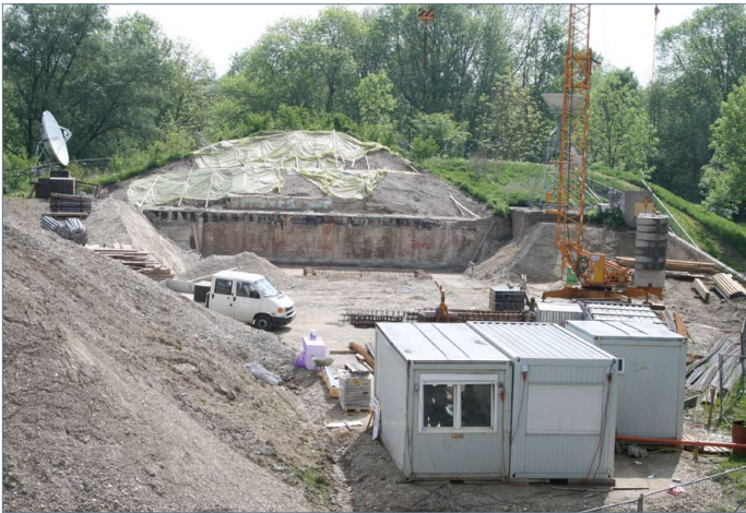
Digging a hole for the new Underground Laboratory
